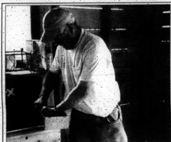
Roger Sterk wiring the Garden House.
