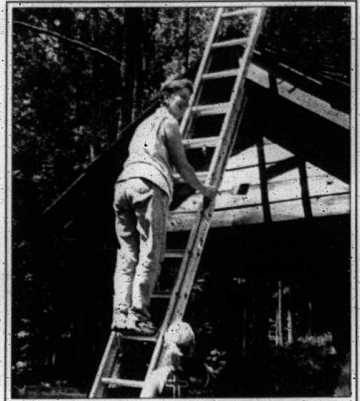
Pam Van Riessen varnishing the covered bridge.
