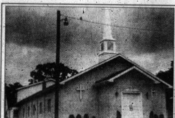
The former Northside Baptist Church building.
