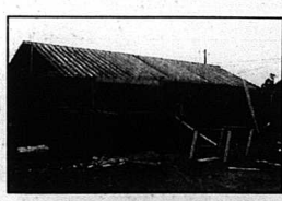
New House Under Construction
