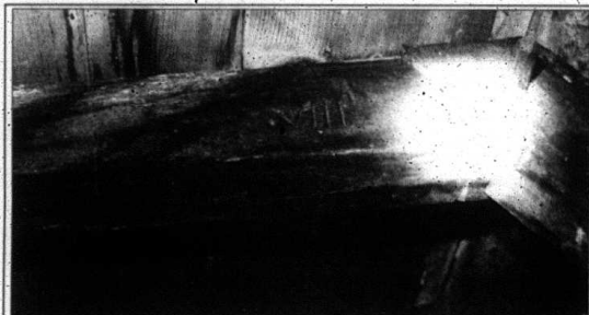
The original Roman numeral markings can still be seen on some of the ceiling beams in the former coach house at Red Hill.
