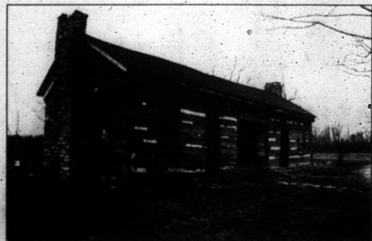
The old coach house at Red Hill is one Rockcastle County's oldest landmarks and is in the process of being restored.
