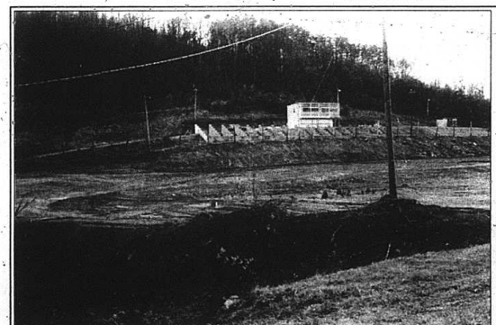
Work is well underway on the new I-75 Speedway, which is open this Spring at Cove Branch. The former Rockcastle Raceway has a full slate of races scheduled for next season.
