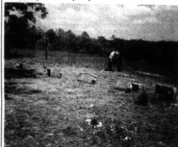
Tommie Falin putting in new fence posts at E.B. Allen Cemetery on Toddy Payne Rd.
