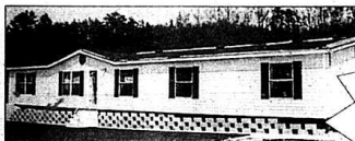
28' Wide Chandelur -Wood wrapped, 5 BR,2 Bath, Big Family Room Fireplace
